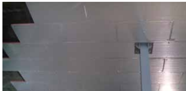
Figure 6 Board joints squared
